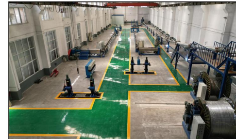
MV Cable Workshop
